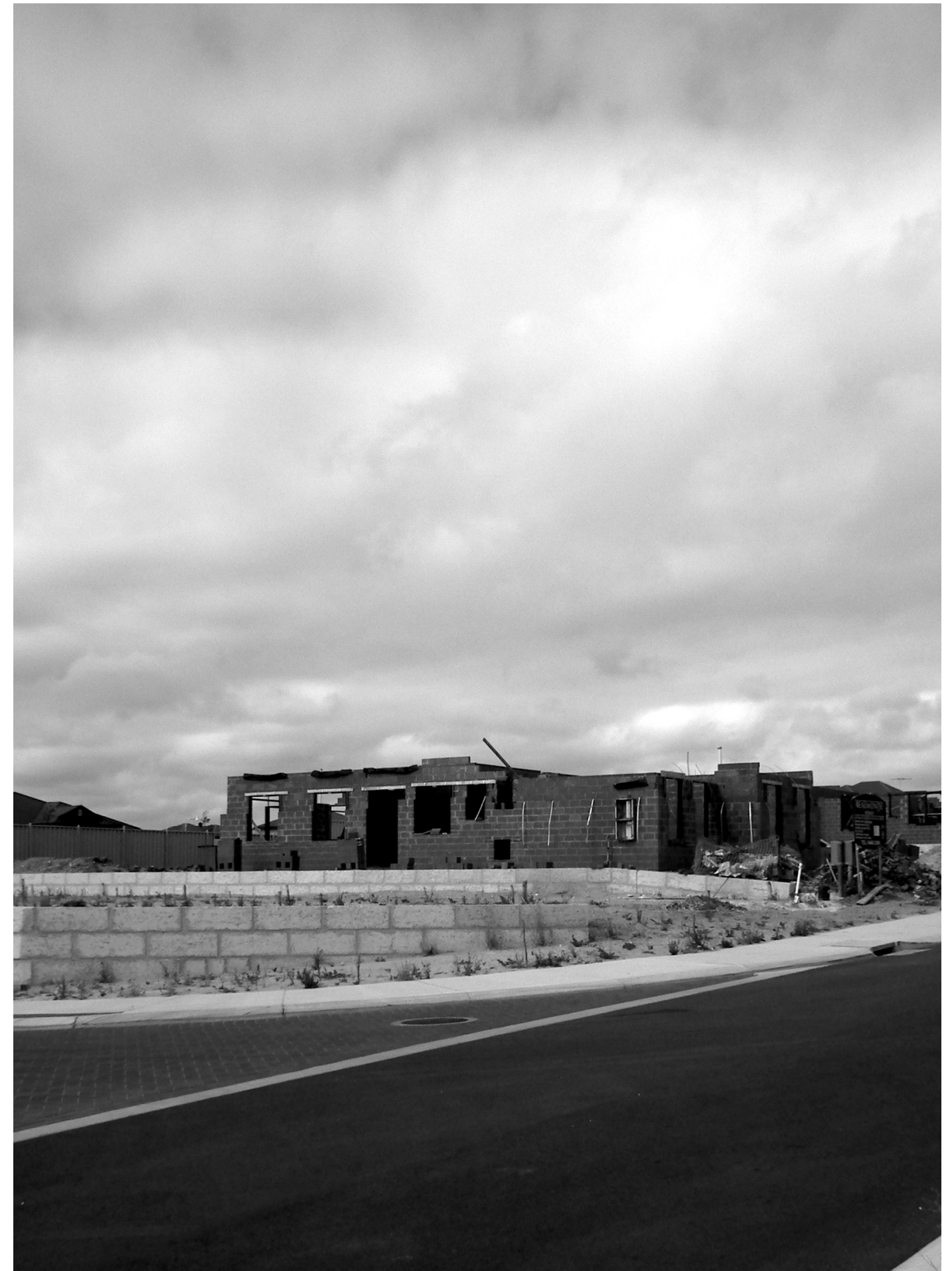
An Ugly New House Under Construction
